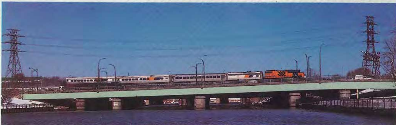
SIX existing highway bridges (but not railway crossing) at Humber River will be replaced in stages.
